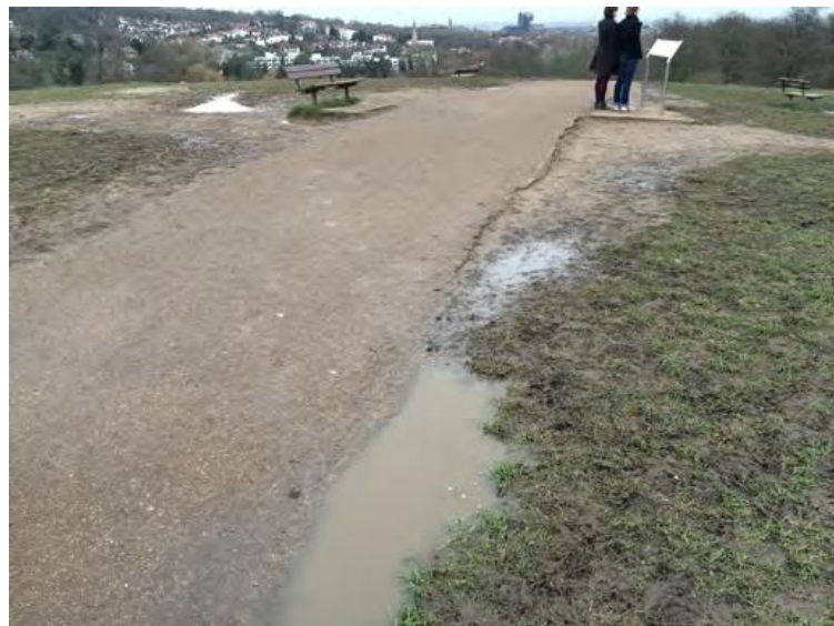
Figure 1: Highest point of Parliament Hill - eroded and deeply compacted
